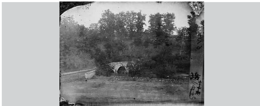
The Lower, or Burnside, Bridge from the Union Side
